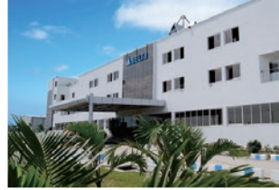
Rudrapur Plant (Green Building)
