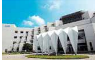
Tainan Plant (Diamond-rated Green Building)
