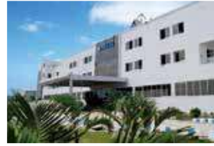
Rudrapur Plant (Green Building)
