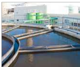
Water & Wastewater Treatment
