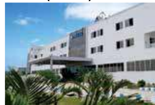
Rudrapur Plant (Green Building)
