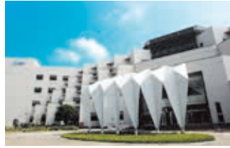
Tainan Plant (Diamond-rated Green Building)
